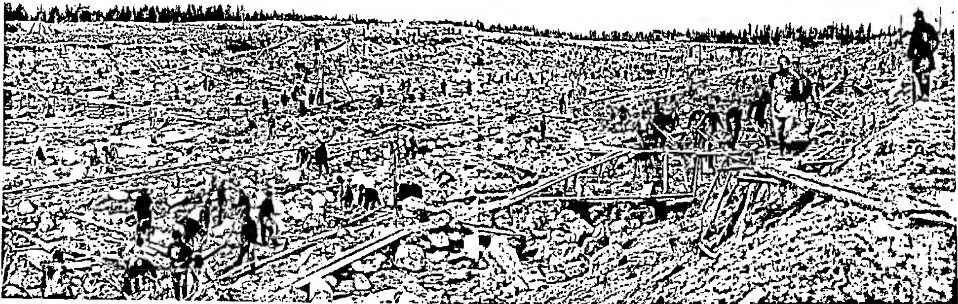
The construction site of the BBK, or Belomorkanal, the canal between the White Sea and the Baltic. This pharaonic project resulted in the deaths of tens of thousands of prisoners in 1932-33. The canal was opened amid great pomp by Stalin and his acolytes but proved to be useless. © Coll. Tomasz Kizny/Vu
